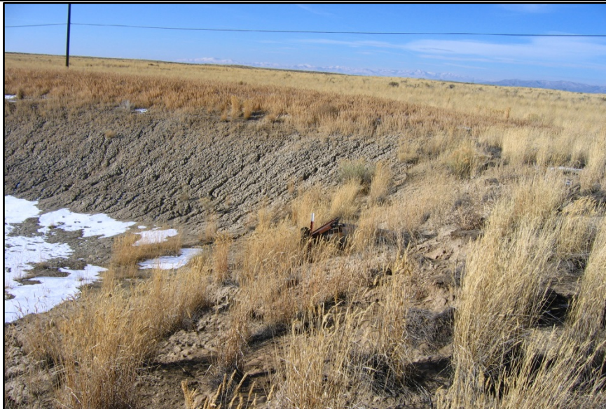
Figure 2. SPERT DISP 3 settling pond and drain inlet.
