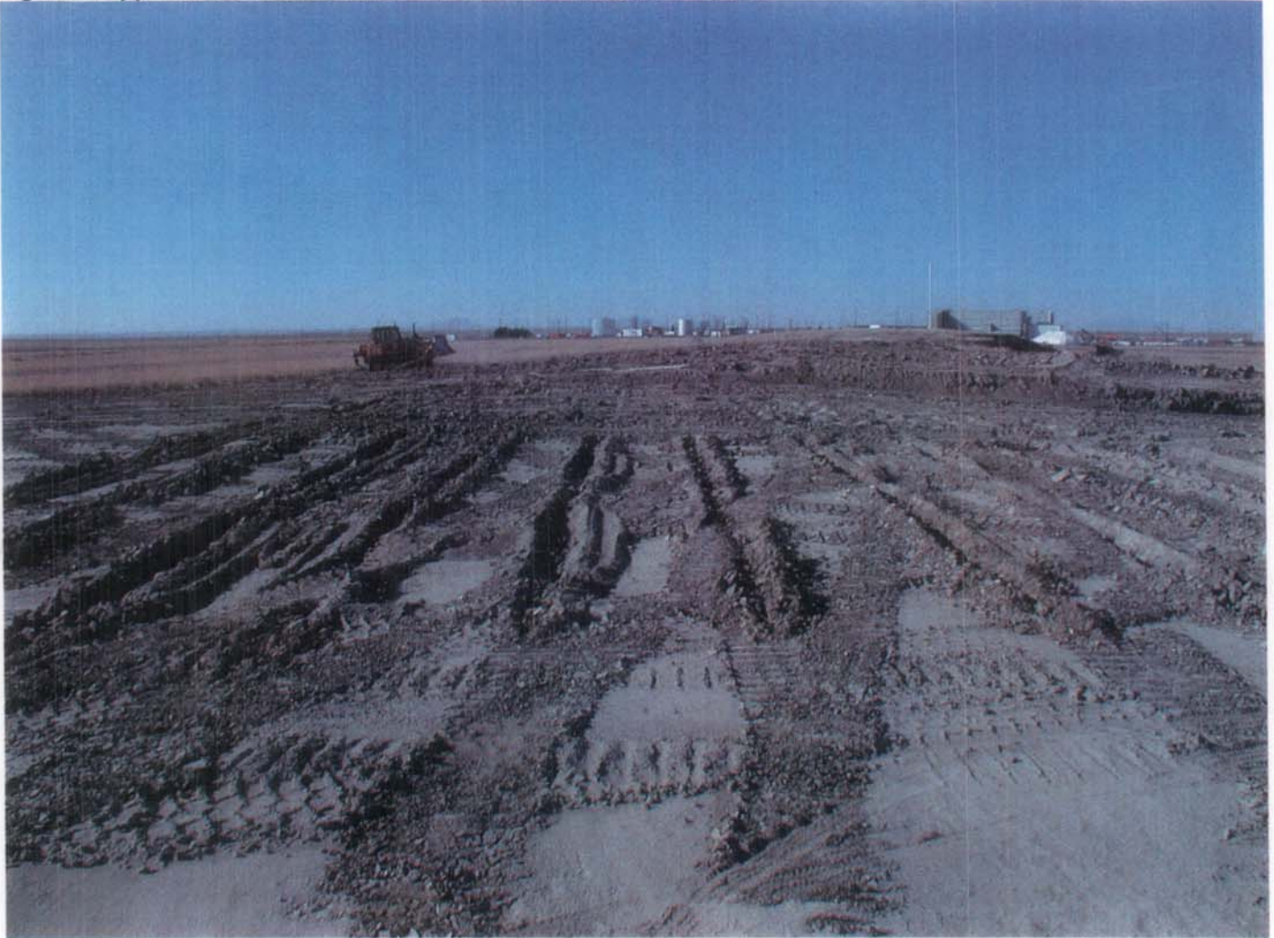
Figure 2, General location of TSF-57 Fuel Line Excavation looking South toward TAN-611.
