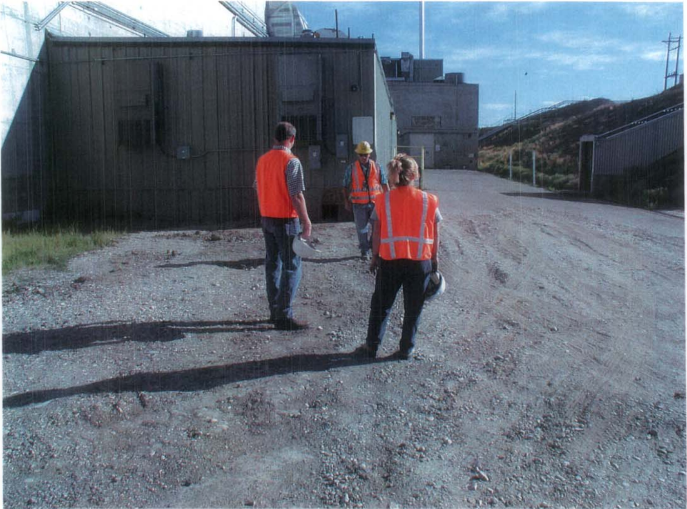
Figure 3, Location of TSF-57 Fuel Line Excavation looking Northeast toward TAN-607 and its Annexes.
